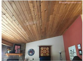
**Photograph 6: Now What? -** Air leaky cathedral ceiling with no access....a scissors truss with a wood board ceiling and limited attic insulation and limited attic ventilation. Beautiful and ugly at the same time.
