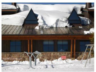
**Photograph 9: Don't You Just Love Aspen –** Top of Ajax...awesome ski lodge. Note the large south facing overhang that traps the heat leading to ice dams and snow slides.
