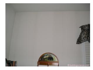
**Photograph 2: Brownian Motion** - "Ghosting" of framing members on the interior gypsum board surfaces of exterior walls.
