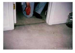
Photograph 1: Carpet as a Filter - Discoloration of carpeting due to particulate accumulation.
