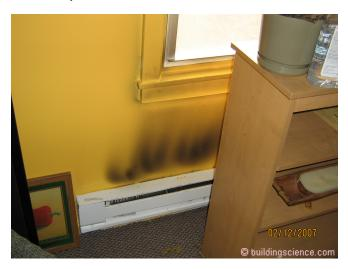
**Photograph 6: Electric Resistance Baseboard Heaters** – What a mess... an energy efficient respirable particle generator.
