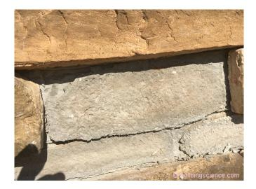
**Photograph 6 - Manufactured Stone Veneer Adhesion Failure:** Bond failure is at the veneer-thin set interface.
