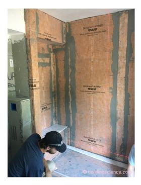
**Photograph 8 – Tile in Shower:** Installation of tile over an impermeable waterproof membrane must be done with unmodified mortar. Evaporation cannot occur through the waterproof membrane into the tile backer board and evaporation cannot occur outwards through the shower tile into the shower area. Therefore, only unmodified thin set can be used. If a modified thin set is used a full bond does not occur.
