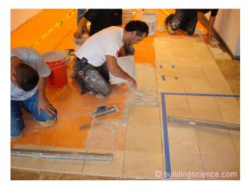
Photograph 7 – Floor Tile: Installation over an impermeable anti-fracture membrane must be done with unmodified thin set. Evaporation or drying cannot occur downwards into the concrete slab through the anti-fracture membrane. Since tiles are also waterproof and vapor closed evaporation or drying cannot occur upwards through the tile. No evaporation. Therefore, only unmodified thin set can be used. If a modified thin set is used a full bond does not occur.
