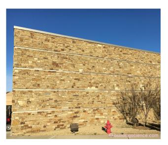
Photograph 4 – More Adhesion Failure: High rainwater exposure.
