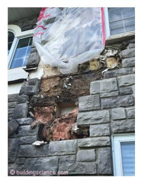
**Photograph 2 – Disaster Made Worse:** Interior plastic vapor barrier preventing inward drying coupled with a 2x6 insulated frame wall reducing energy flow thereby further reducing drying.
