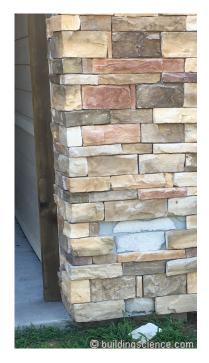
Photograph 3 - Adhesion Failure: High rainwater exposure.
