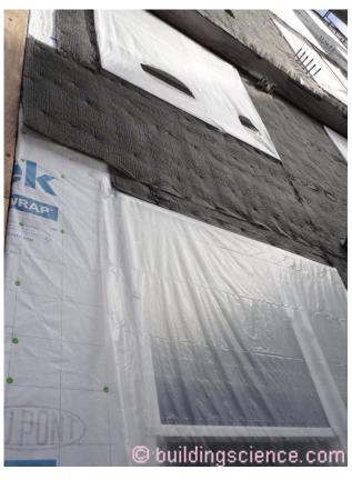
**Photograph 8: Drainage Mat** – Drainage and hygric redistribution for a stucco assembly is provided by a drainage mat installed over a mechanically attached WRB installed over exterior gypsum sheathing.
