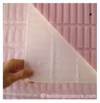
**Photograph 7: Filter Fabric and Channels** – Channels cut into extruded polystyrene (XPS) coupled with a filter fabric to exclude mortar droppings or to prevent the base coat of stucco from inhibiting drainage.
