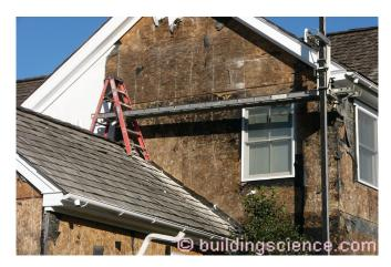
**Photograph 2: Stucco Failure** – Not a pretty sight. No drainage coupled with moisture sensitive sheathing (oriented strand board – OSB) and high levels of thermal resistance (not enough energy flow to facilitate drying).
