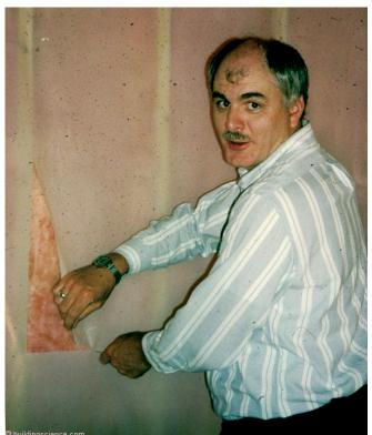
Photograph 7: What is That Smell? – A very young (at the time) Professor Pat Huelman finding mold and water damage behind a leaking basement foundation wall insulated on the interior with fiberglass batts and a polyethylene vapor barrier.
