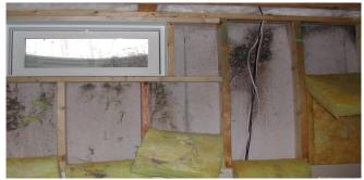
**Photograph 2: More Basement Water Damage** – Notice the ground water "mustaching" at the bottom of the basement window corners. Ah, shafted again...
