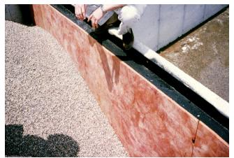
**Photograph 6: More Draining Insulation** – Notice the black dampproofing. This was a very conservative approach....and necessary with low thermal resistance levels of draining insulation. The insulation basically provided only the drainage function and the capillary break. The vapor control function was provided by the dampproofing.
