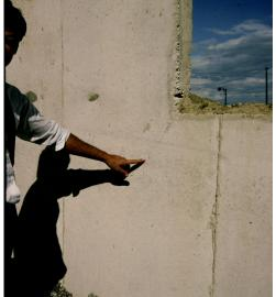
**Photograph 3: Concrete Crack** – Cracking typically happens at stress concentrations such as at punched openings. The hand pointing to the crack belongs to a young (at the time) James Lischkoff...before he became a famous Canadian building scientist.
