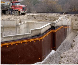
**Photograph 4: Drainage Mat** – An airgap is provided by "bumps" or "dimples" in the membrane. The airgap provides drainage controlling hydrostatic pressure.
