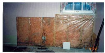
**Photograph 1: Basement Water Damage** – Insulating and finishing a basement on the interior that is experiencing ground water leakage often leads to significant damage.
