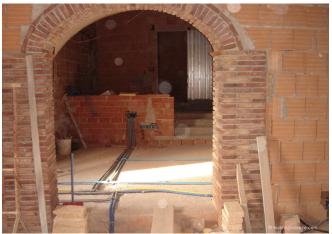
**Photograph 15: Services -** The services are run in the floor slabs and on the walls they are cut into the terracotta blocks.
