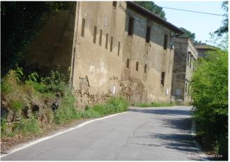
**Photograph 2: Abandoned Buildings -** Surprisingly many buildings are abandoned and in disrepair. Spalling of renderings is typical. Rainwater management is poor. Flashings are non-existent.
