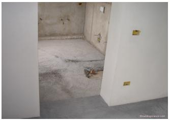
**Photograph 17: Topping Slabs** – Topping slabs are cast over the top of the services to provide a base for floor finishes.
