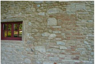
**Photograph 9: Exterior Stone -** The exterior stone is fastidiously pointed and repointed with lime based mortar. Notice the random intermittent use of thin terracotta bricks in the exterior layer...they sure know "style" in Italy. Water entry is controlled by rain shedding, storage absorption and redistribution. The lime based mortar is sacrificial.
