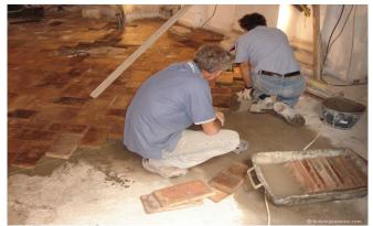
**Photograph 18: Terracotta Tile Floor Finish -** Notice how the terracotta tile is pre-wetted to prevent desiccation of the setting bed. The concrete surface is "shot blasted" or "scarified" and a non-polymer modified cement is used to set the terracotta tile.
