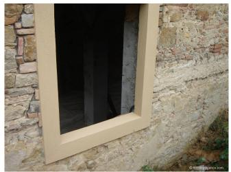
Photograph 14: Concrete Lined Punched Opening - The big change in recent time is to line the openings with concrete which is a huge improvement...a Tuscan version of "fluid applied flashing". Not bad.....but... they often set the window or door behind the concrete lining instead of over top of the concrete lining resulting in a "reverse flash".
