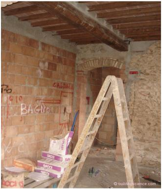
**Photograph 8: Tuscan Wall -** A stone layer on the exterior is supported on the interior by terracotta blocks and bricks. There are no voids. This is a classic "mass" wall not a veneer or cavity wall.
