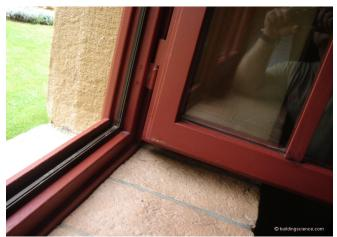
**Photograph 11: Window Opening -** Tuscan openings we get no flashing. None.
