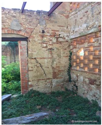
Photograph 4: Wall Assembly - Miss-mash of brick and stones and clay blocks.
