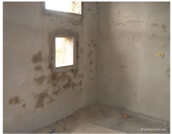
**Photograph 10: Lime Plaster -** The interior lining of exterior walls is a lime based plaster.
