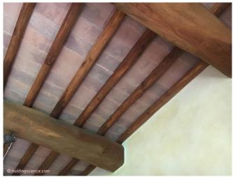
**Photograph 6: Tuscan Roofs -** Terracotta bricks supported by wood rafters and wood timber beams.
