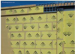
Photograph 2: More New Systems – Gypsum board sheets covered with trowel applied membrane.
