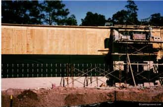
**Photograph 5: Old School** - Apparently a point missed by folks is that we installed asphalt impregnated felt, Type D coated building papers and building wraps by nailing and stapling them and then we nailed and screwed cladding systems through them and did nothing special at the resulting penetrations and the world did not come to an end....
