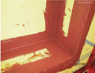
Photograph 8: Reinforced Joint - Liquid applied membrane reinforced with mesh.
