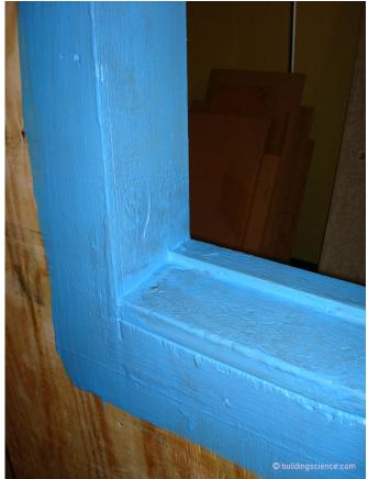
**Photograph 4: Window Opening** – Lots of joints and inside and outside corners. How we deal with the joints and the inside and outside corners is the trick. Note the "filet" sealant in the "end dam" and "back dam" under the liquid applied membrane.
