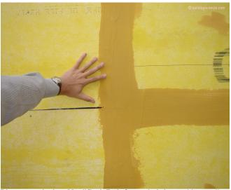
Photograph 9: Modified Reinforced Joint – No sealing filling the joint...only mesh reinforcing.
