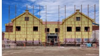
Photograph 3: Still More New Systems - Sheet goods with integral water and air control layers.
