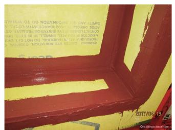
**Photograph 6: Stress Reduction -** So how to reduce the stress on the liquid applied membrane? Easy. Fill the joint with a sealant. Big improvement in performance. This works big time in corners. With inside corners a "filet" bead yields a nice curve rather than sharp change in direction.
