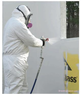
**Photograph 1: New Systems -** The trend is to sheet goods covered with spray applied liquid membranes. Note the word "sheet goods".
