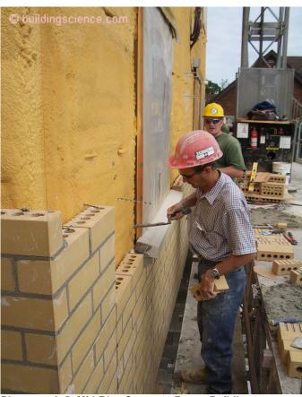
**Photograph 5: Mid-Rise Concrete Frame Building** – Masonry back up wall with a 3-inch layer of 2 lb/ft3 density spray polyurethane foam (SPF). The SPF is the continuous insulation layer – and is fire resistant but still combustible. The cladding is a non-combustible brick veneer over a ½ inch air space. This assembly has passed the NFPA 285 test.
