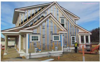
**Photograph 6: Low-Rise Wood Frame Building** – This is the NIST Net Zero Energy Test House. The continuous insulation layer is 4 inches of foil-faced iscocyanurate. The cladding is non-combustible fiber cement siding installed over 1x4 wood furring (3/4-inch air space). This assembly is not required to pass the NFPA 285 test and would easily outperform the Grenfell Tower in a fire because of the fiber cement cladding and the small "rain screen" airspace (3/4 inch)."
