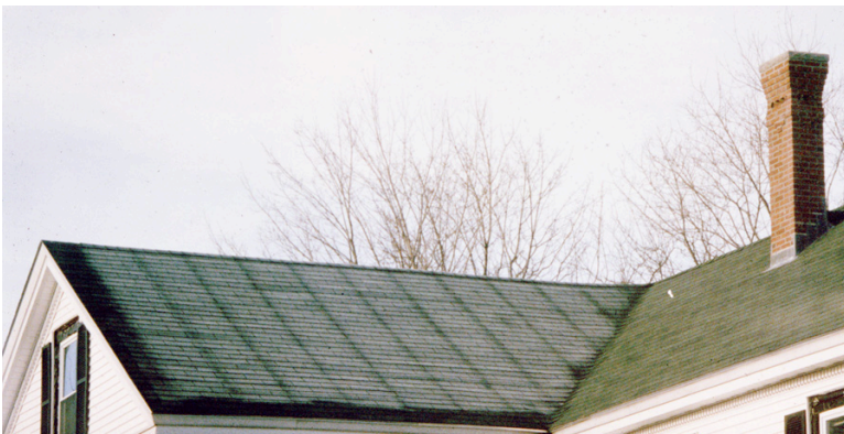
Photograph 4: Thermal Bridging – Don't need no stinkin infra-red camera. Ouch. Only invited friends over at night so I wouldn't be embarrassed.
