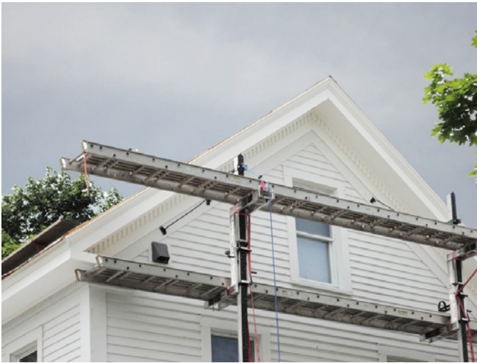
Photograph 9 (above left): Trim Installed —Dentil molding, crown molding and double frieze board done. Note that a second frieze board is installed catching the top edge of the original frieze board. Double frieze boards are not uncommon in New England so that the second frieze board does not look out of place. This approach allows us to leave the original frieze boards in place along with not having to remove and reconstruct the gable siding. Next step stainless steel drip edges and shingles.
