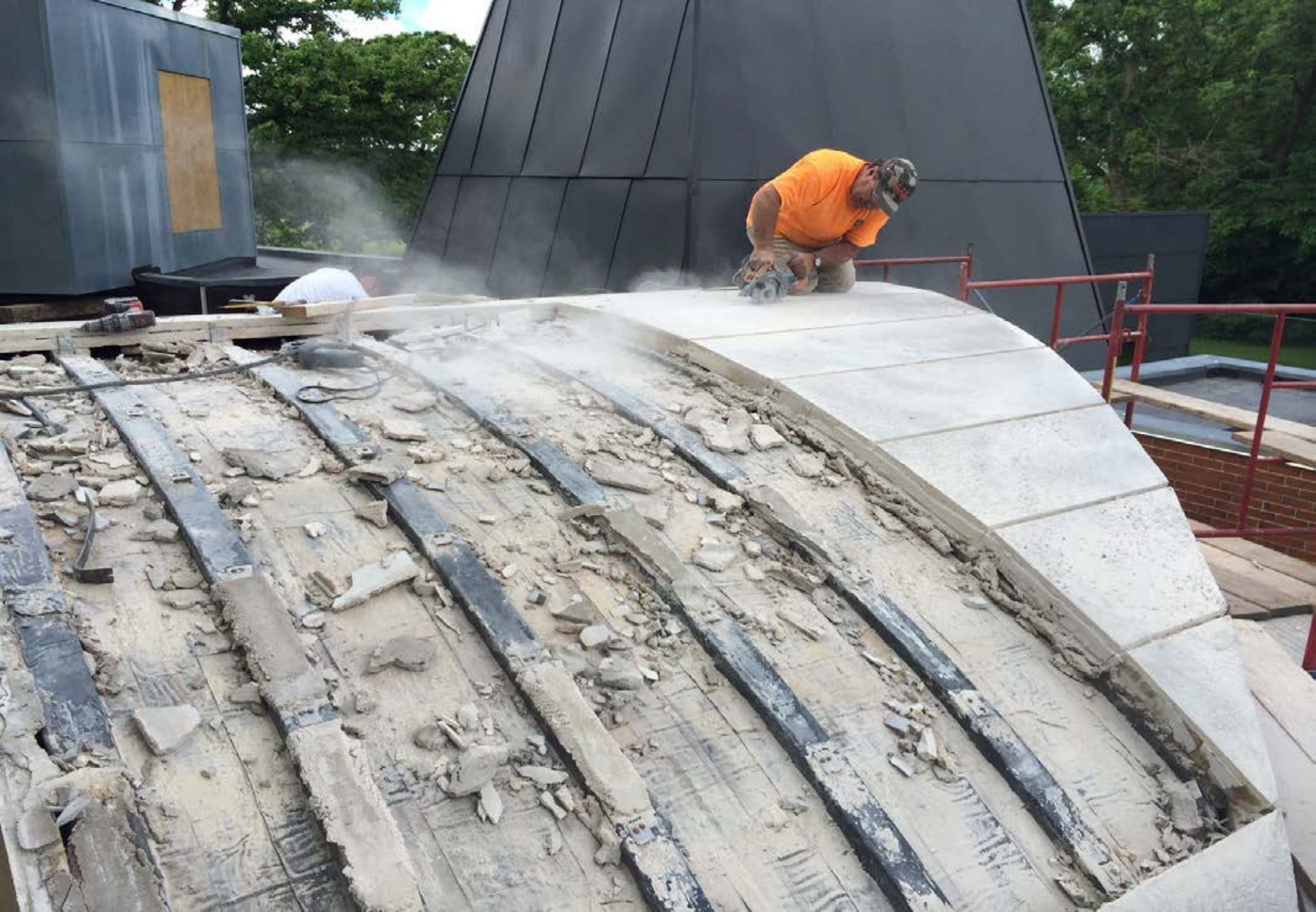
Winton House | Remove & Re-Install
