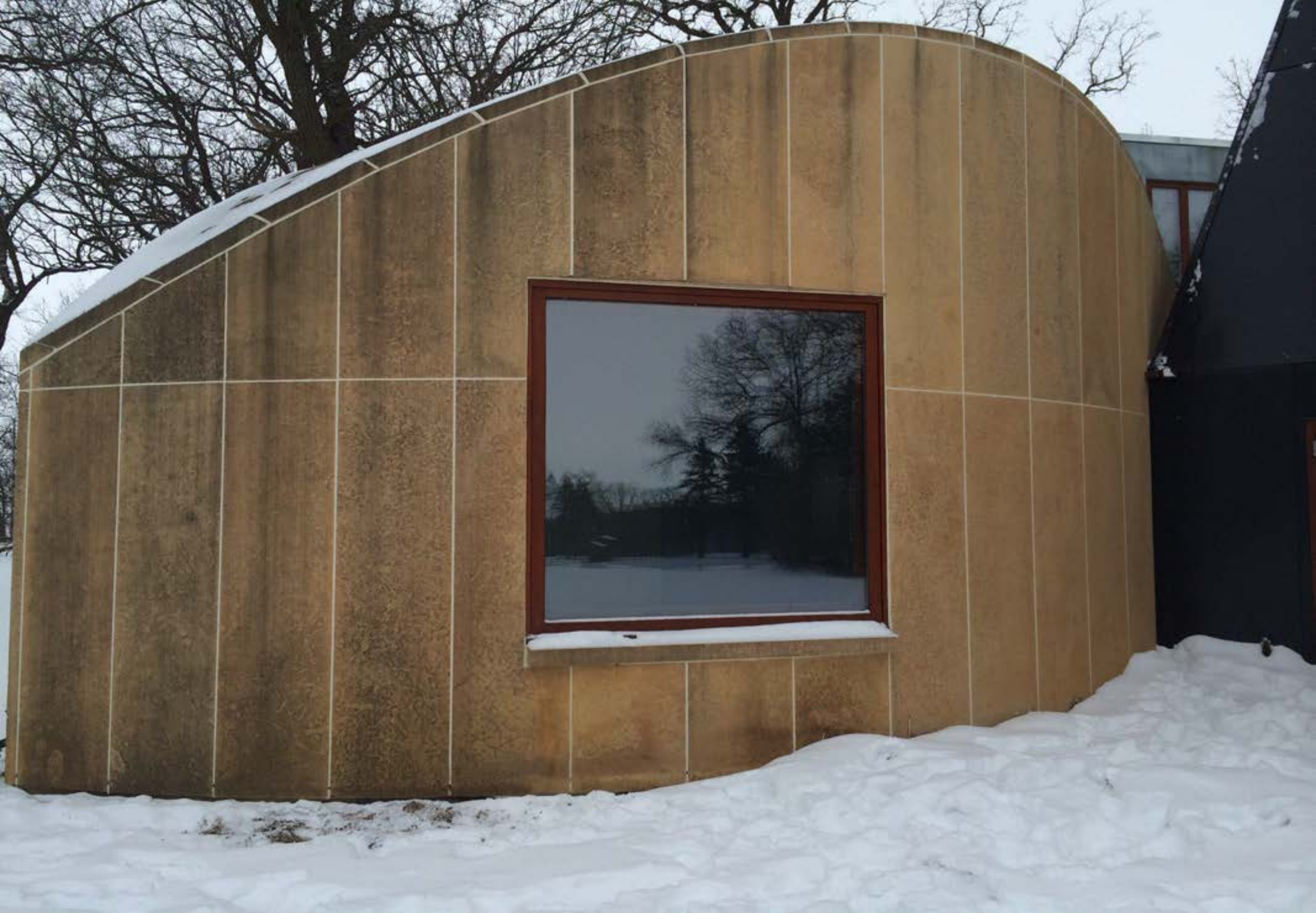
Winton House | Remove & Re-Install
