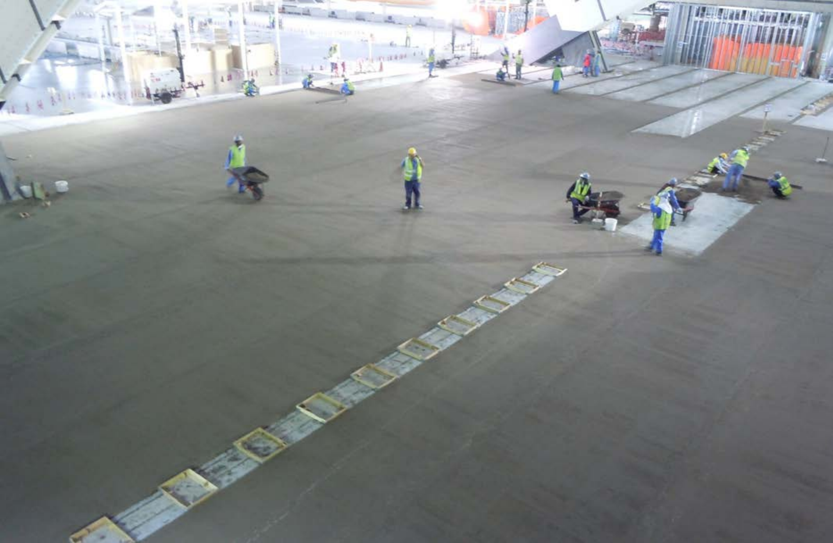
Mortar Screed - Epoxy & Sand
