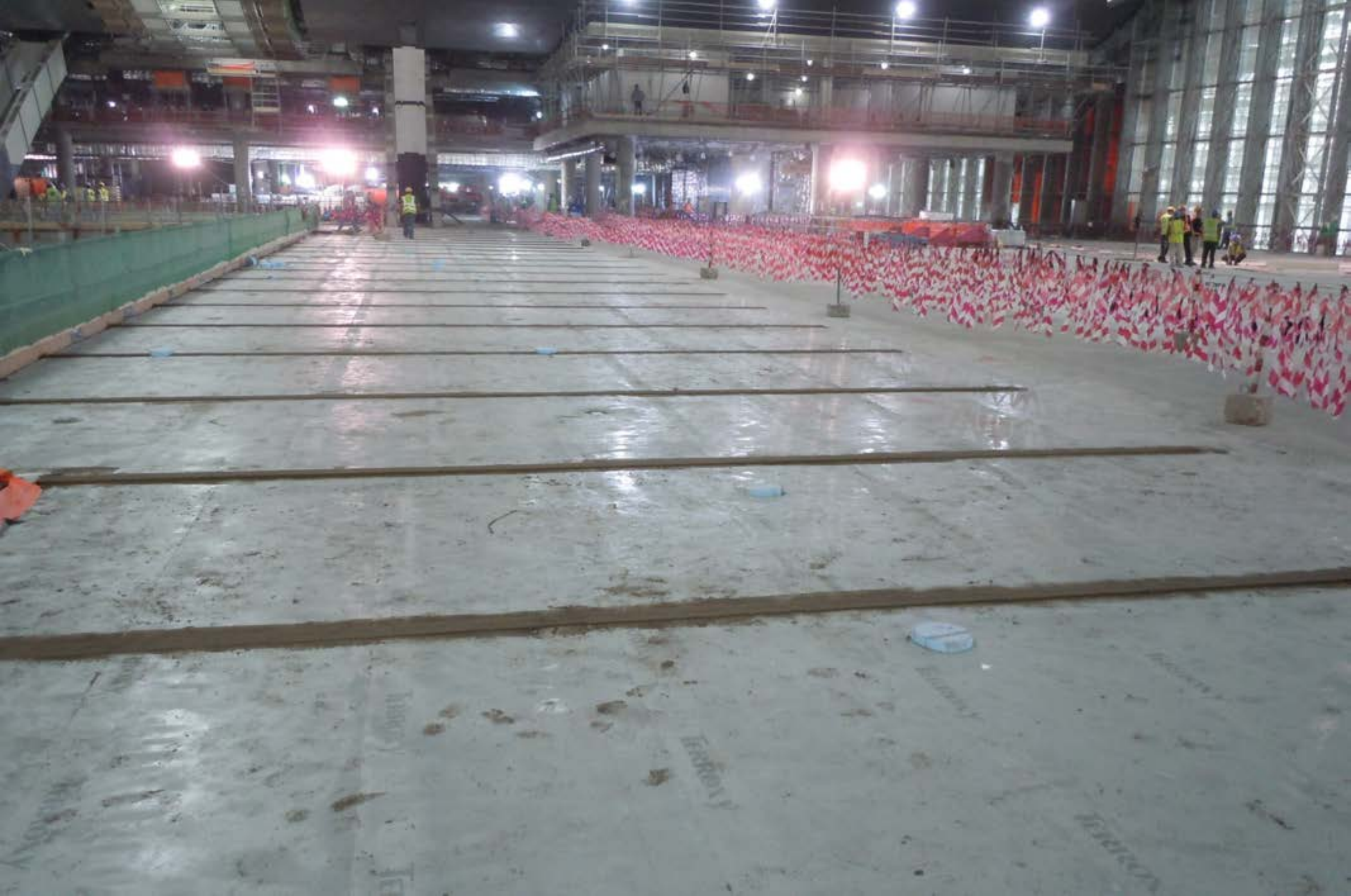
Mortar Screed Rails
