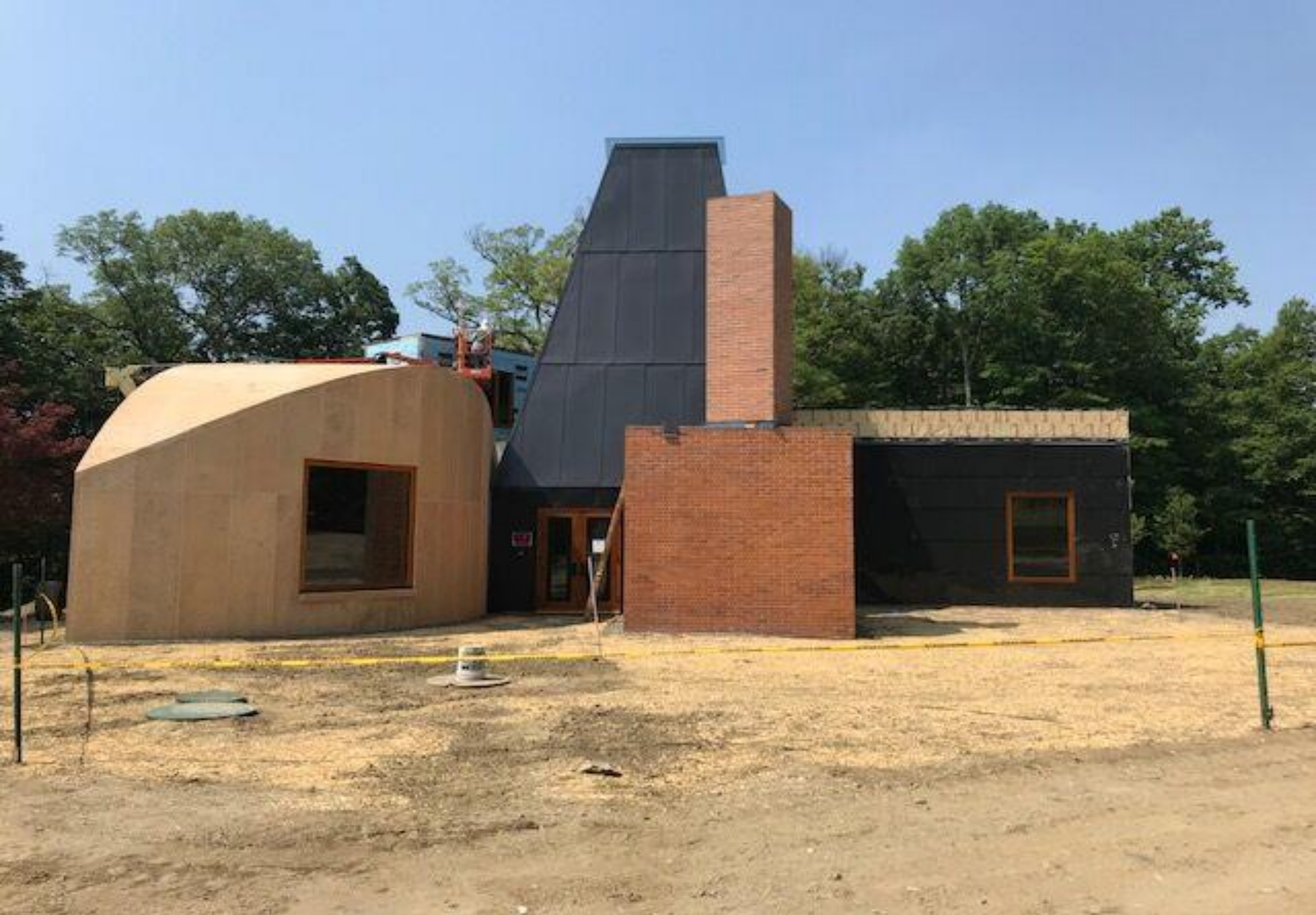
Winton House | Remove & Re-Install
