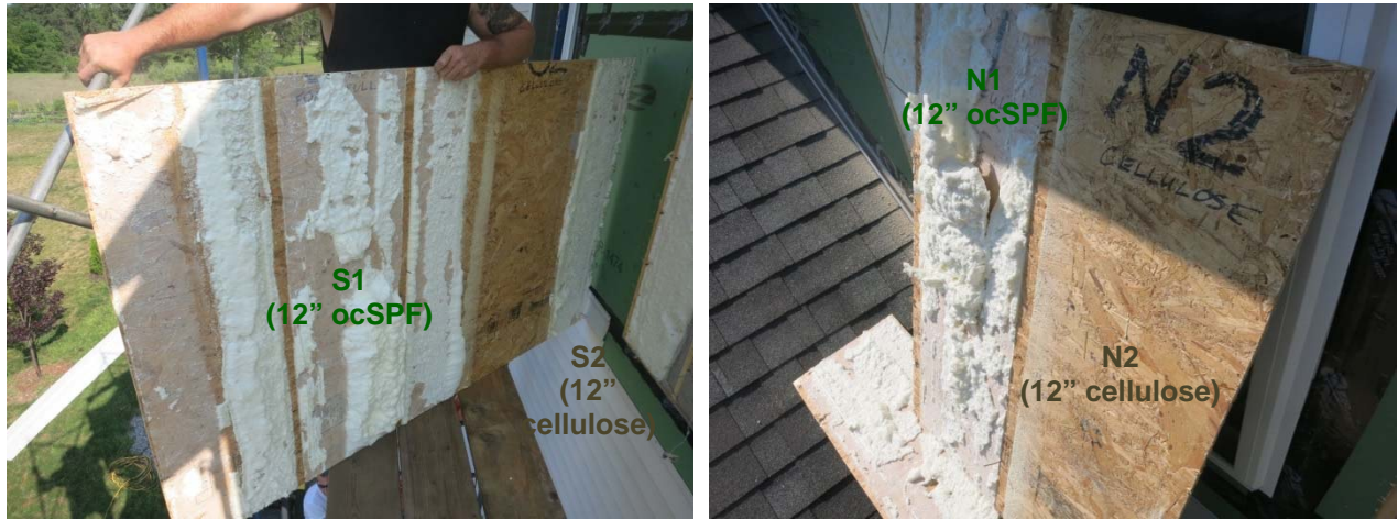
Figure 15: Sheathing conditions at south (left) and north (right)-facing walls
