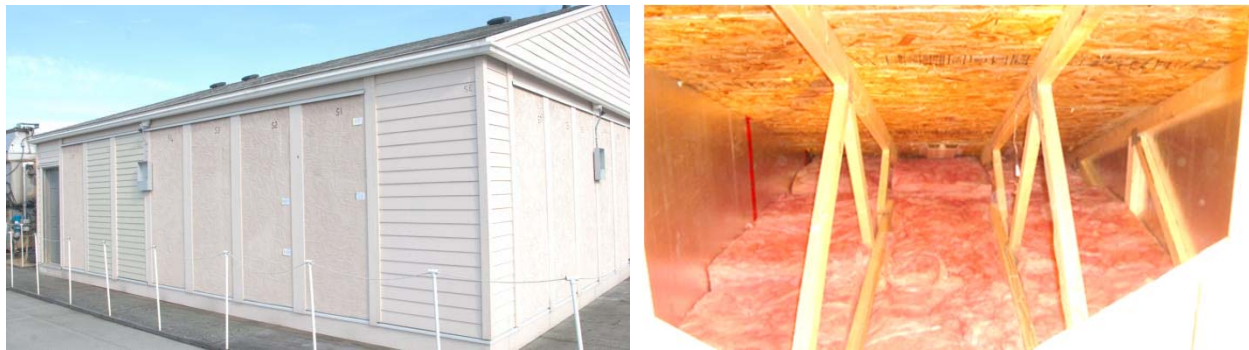
Figure 19: Coquitlam test facility (left), and vented attic
