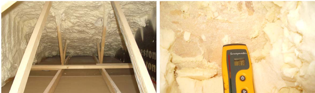
Figure 22: Unvented cathedralized attic in Coquitlam test facility, and sheathing MC measurement
