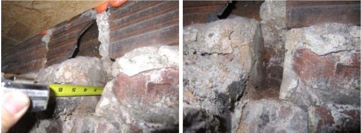
Figure 35. Conditions in joist pocket at north-facing building at addition
