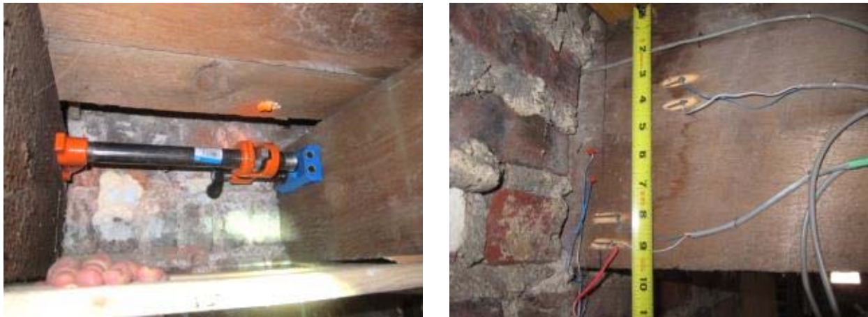
Figure 32. Pocket hole jig (left); installed MC pins (right)
