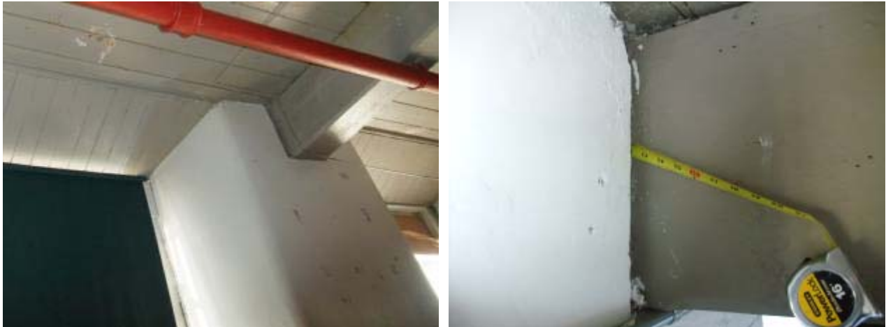
Figure 7. Beam pocket gap on sides; conditions vary by building
