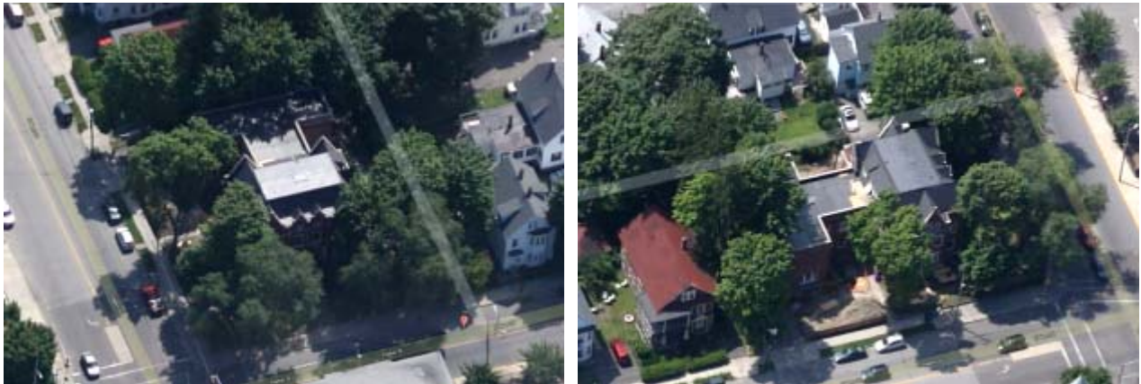
Figure 14. Overhead view of retrofit building from west (left); overhead view from north (right)
