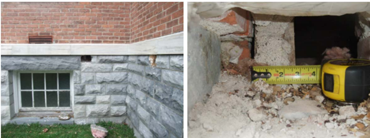
Figure 10. Embedded joist end from exterior showing dimensions and fire cut
