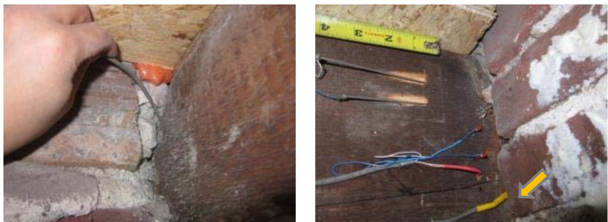
Figure 34. Installation of pocket RH sensor (left); installed RH sensor (right)
