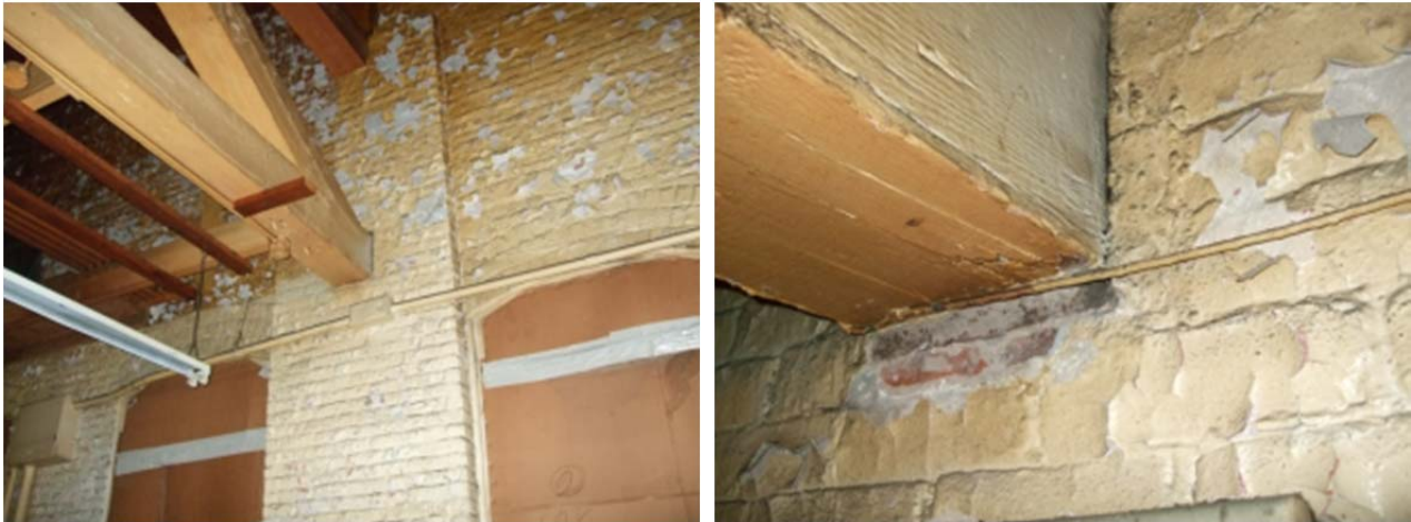
Figure 6. Large timber beam pocket (left); iron or steel bearing plate (right)
