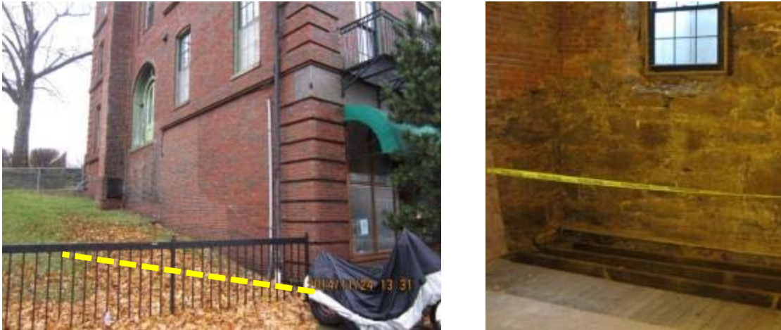
Figure 11. Building exterior grade condition (left); beam interface to below-grade wall (right)
