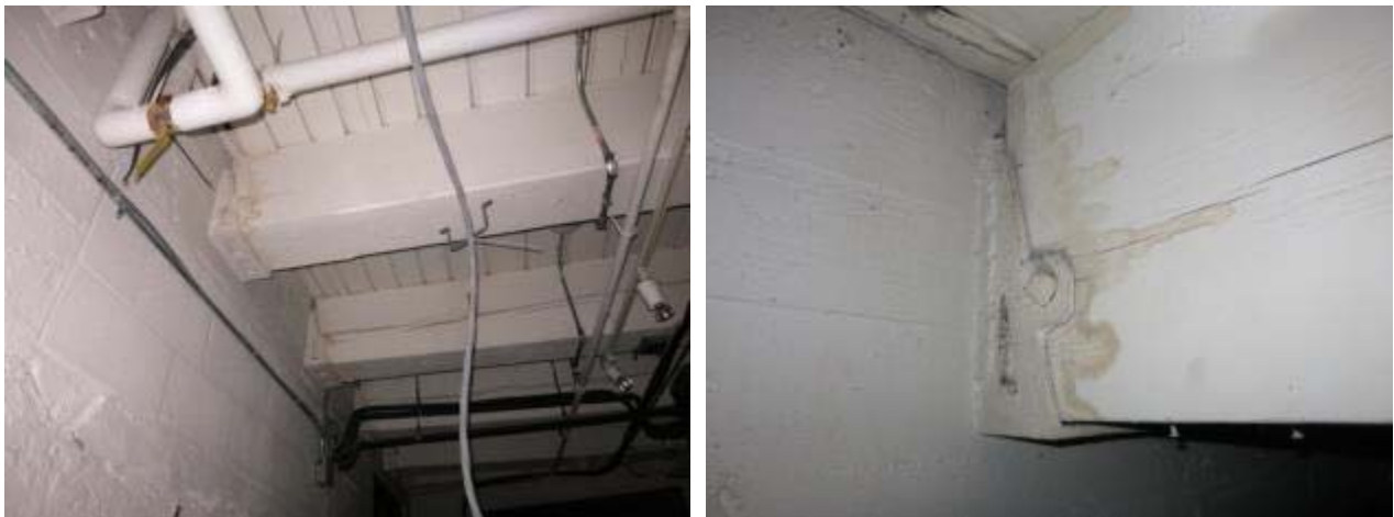
Figure 8. Steel saddle hanger detail, with beam clear of masonry wall at grade
