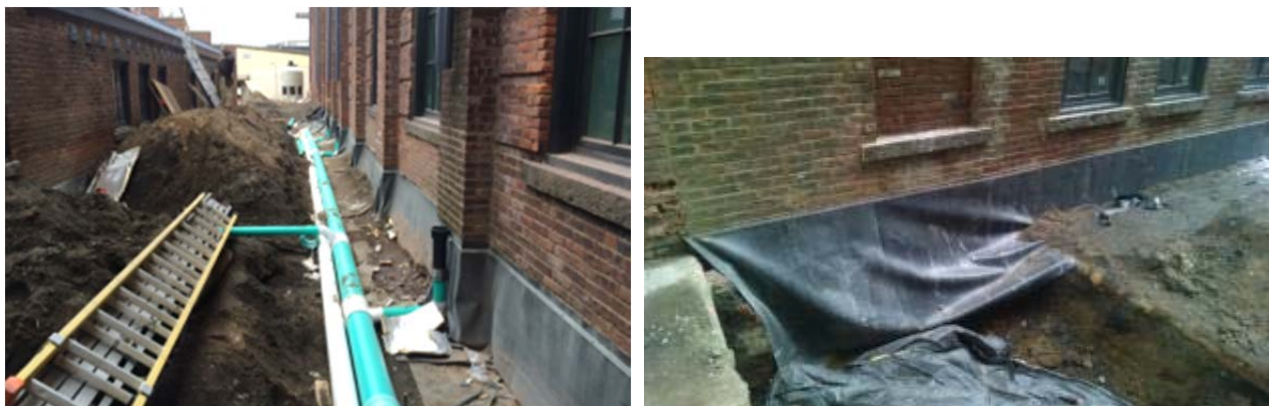
Figure 69. Exterior excavation of masonry building with water shedding detail below grade
