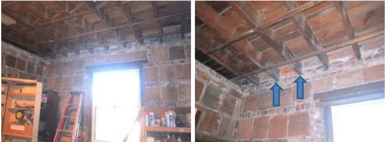
Figure 27. FIRST-N joists showing brick and clay block wall construction
