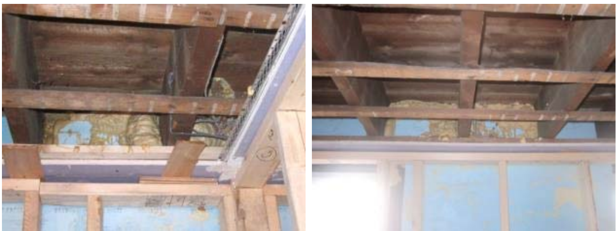
Figure 29. Two-component spray foam air seal at joists BSMT-W1 and BSMT-E1
