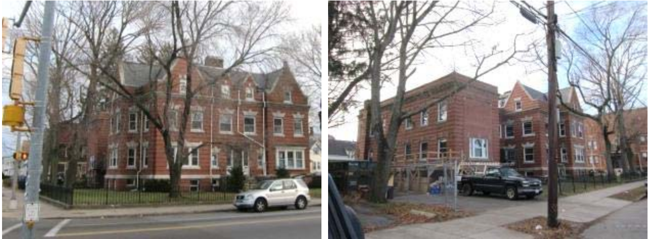
Figure 13. Retrofit building exterior view from west (left); view from north (right)
