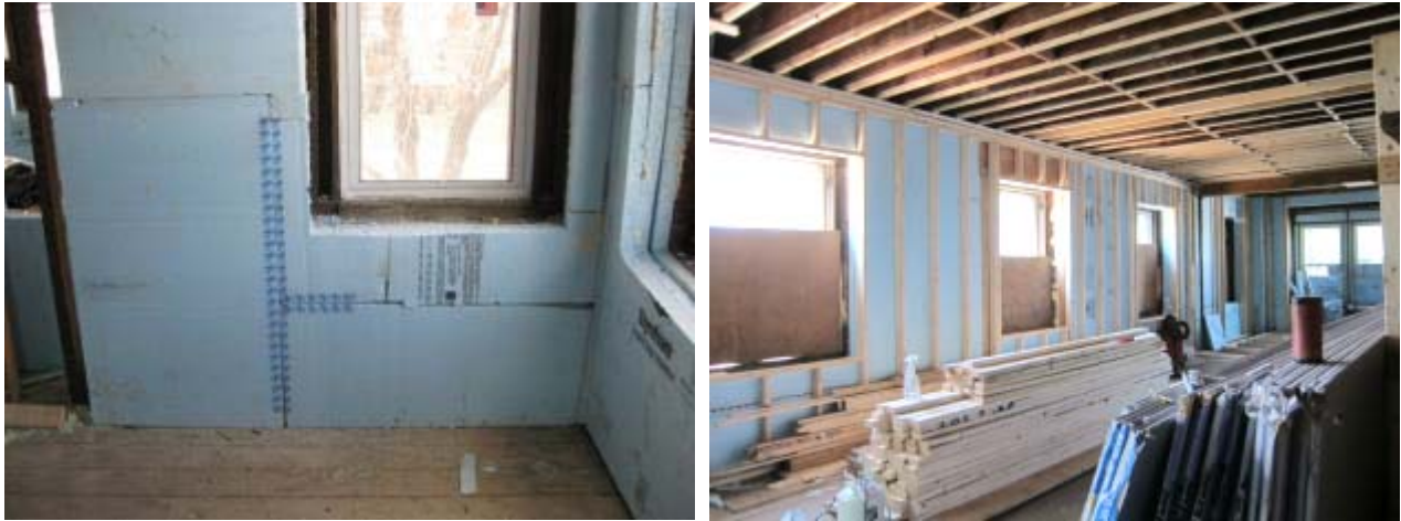
Figure 18. Multiple layers of insulation (left); framing installed inboard of insulation (right)
