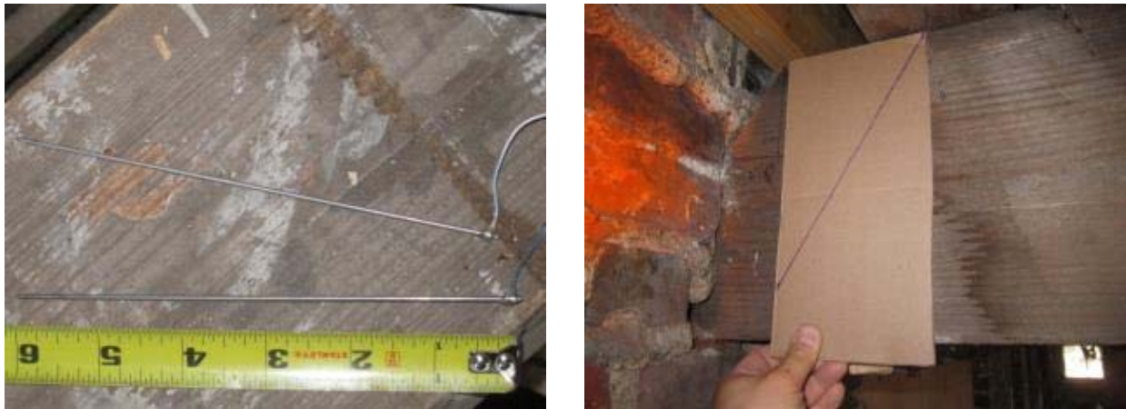
Figure 31. 6-in. extended MC pins (left); determining drilling depth (right)
