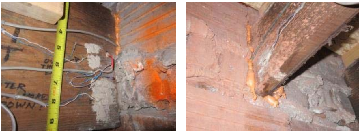
Figure 33. Caulked pocket holes (left); air seal at joist pocket (right)
