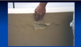
**Problem:** Peeling coating **Solution:** Locate the water intrusion, remove all loose coating, then coat with a product that has superior moisture vapor permeability
