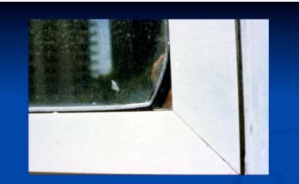
**Problem**: Gasket shrinkage **Solution**: Remove gasket and provide a continuous fillet wet seal joint
