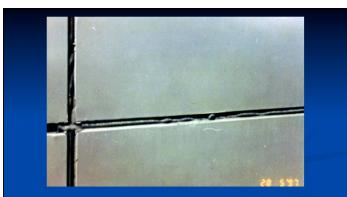
**Problem:** Movement during cure **Solution:** Use open cell BR to speed cure and keep sealant depth at 1/8" to 1/4"
