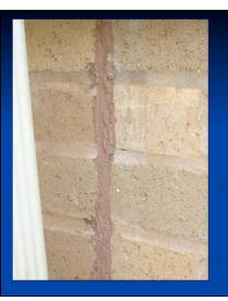
**Problem:** Poorly tooled joint – sealant has not wet out sides of joint
