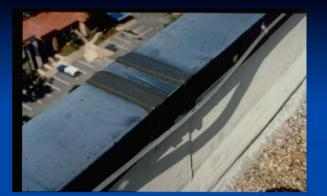
**Problem:** Leaking Parapet **Solution:** Pre-cured silicone adhered with wet sealant
