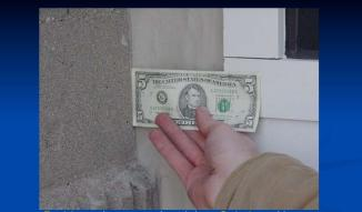
**Problem:** Large sealant joint. Solution: Not a problem if the sealant depth is ½" or less. Requires significant applicator skill. Choice of backer is important.
