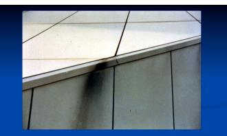
Problem: Dirt rundownSolution: None withcurrent design – Water must be channeled away fromthe face of the panel
