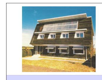
Saskatchewan Conservation House – 1977 R-40 double stud walls R-60 ceiling Triple glazed windows Air to air heat exchanger 0.8 ach@50 Pa Leger House - USA - 1977
