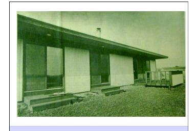
Lo Cal House - USA – 1976 Wayne Shick and Bud Konzo R-30 double stud walls R-30 vented roof Triple glazed windows Air to air heat exchanger Double Wall Patented in US - 1976 Richard Bentley patent discusses airtightness and air-to-air heat exchangers
