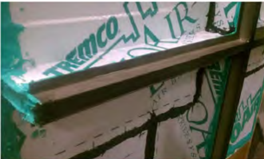
Close-up of panel joint
