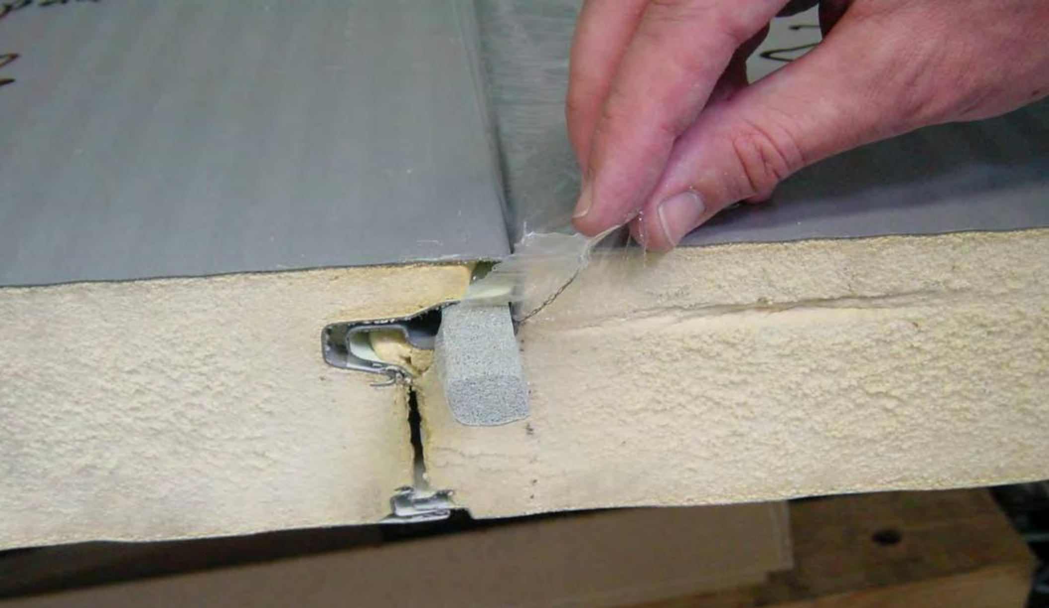
SIP Panel Installation/ Fabrication
