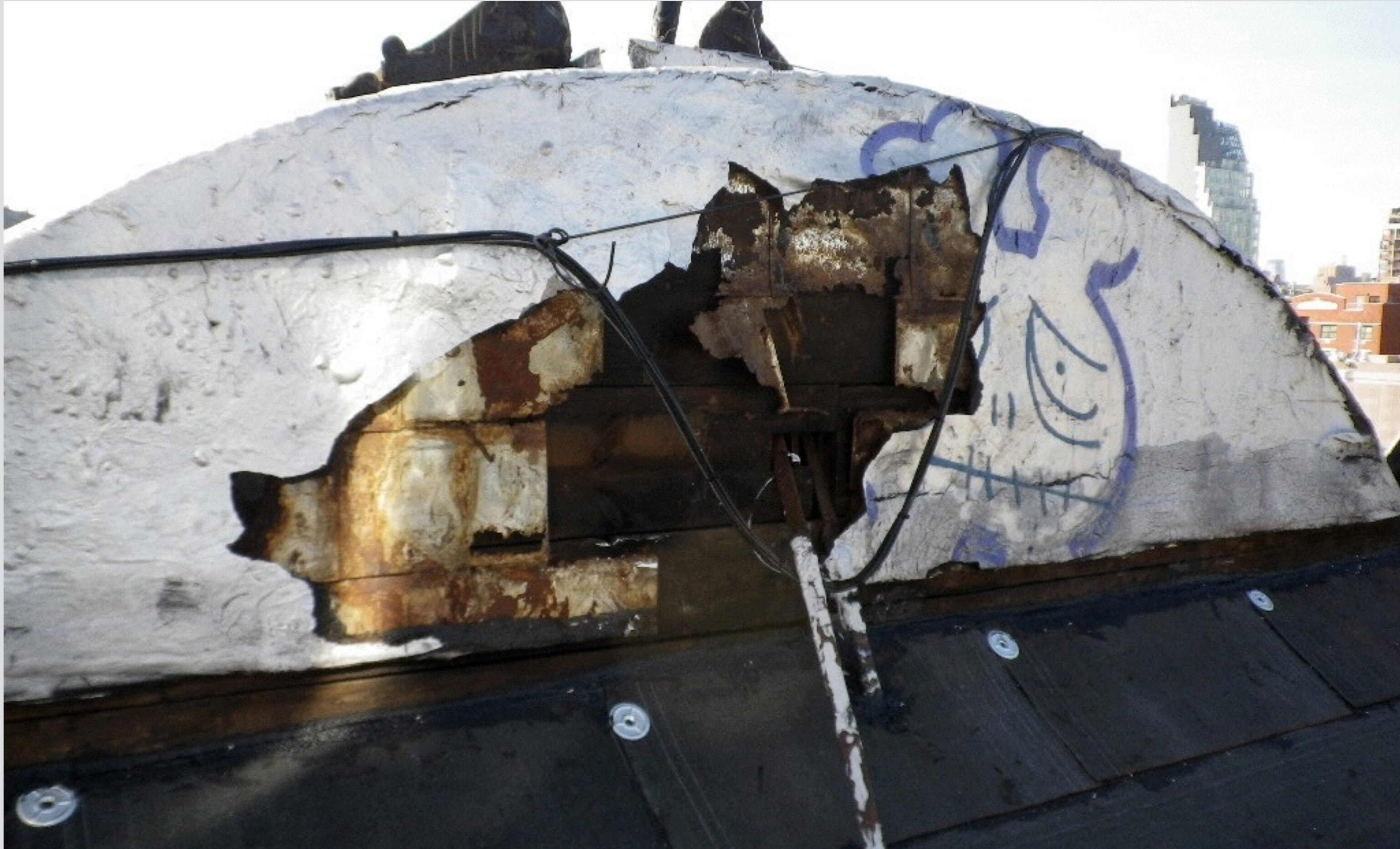
Rear of cornice covered with flashing cement
