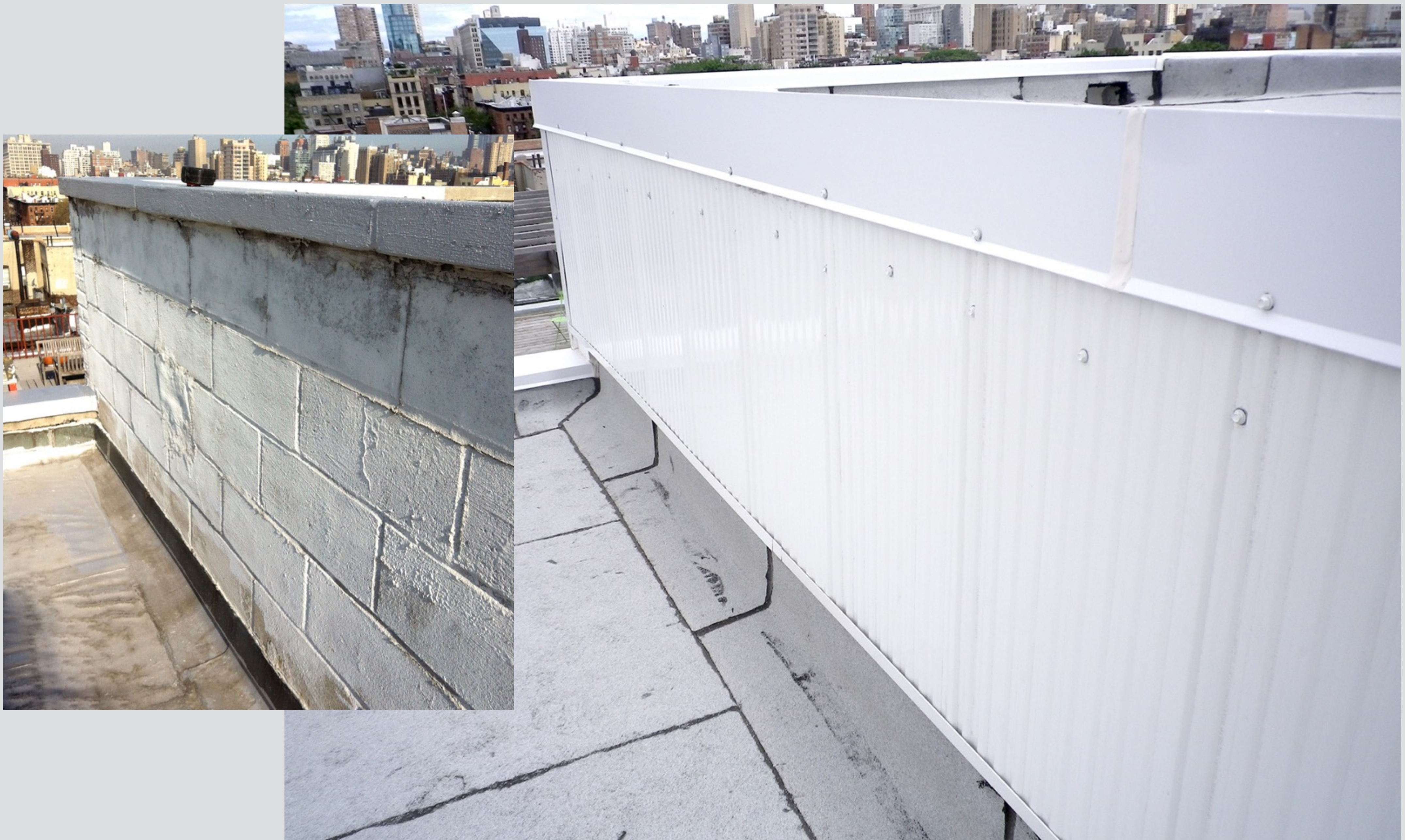
3"XPS on walls, 6" XPS on deck, Elevator service calls eliminated. XXXX
