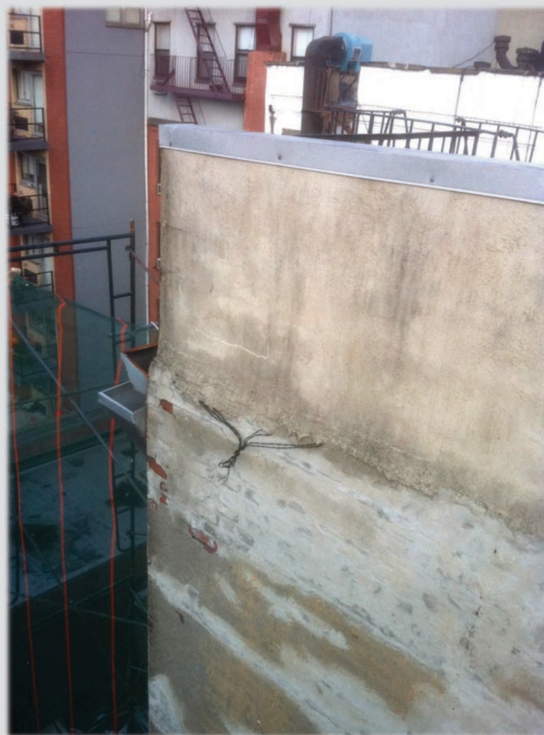
1996 hollow CMU parapet replaced original solid brick parapet
