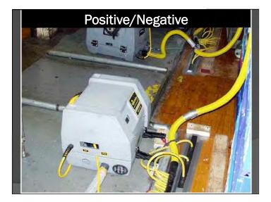
The power of suction pulled newly poured concrete through a studded wall, flooring flutes, and up through drying holes, through hoses and into the blower
